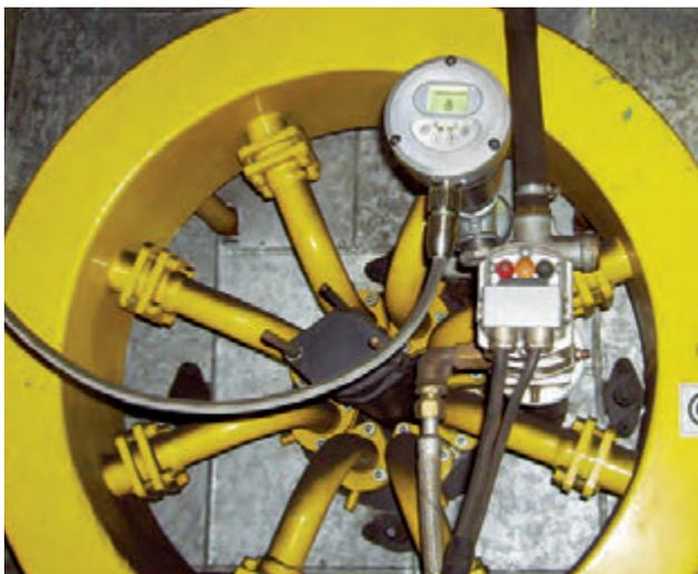
LAMTEC flame monitoring system F300K in action.
