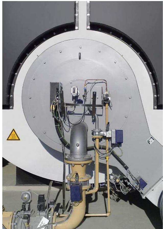
The set fuel/air curves can be shifted using two correction inputs for disturbance variable feedforward during operation. As such, this can help to offset influences on combustion, e.g. changes to the suction air temperature.
