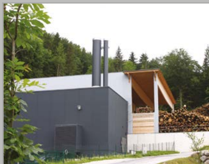
Image: Heating plant in Fuschl am See
